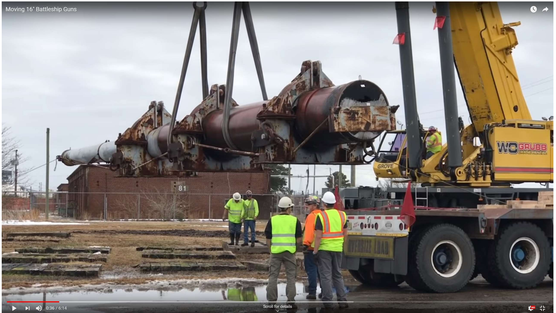
16-inch/50 barrel on the move at St. Juliens Creek Annex
