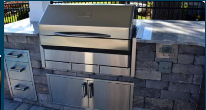
Outdoor Kitchen Installation
