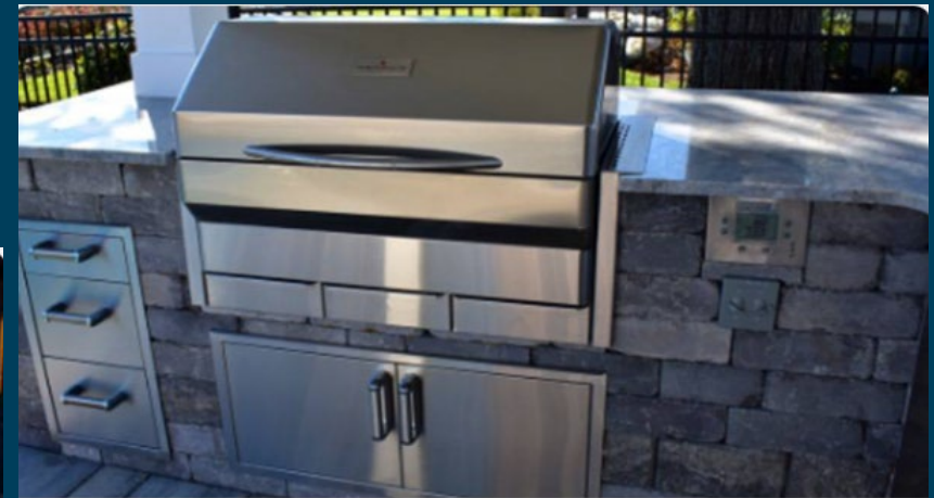
Outdoor Kitchen Installation
